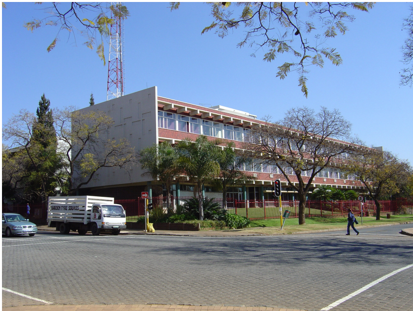
Fig 15. View of fire station across Bosman Street
