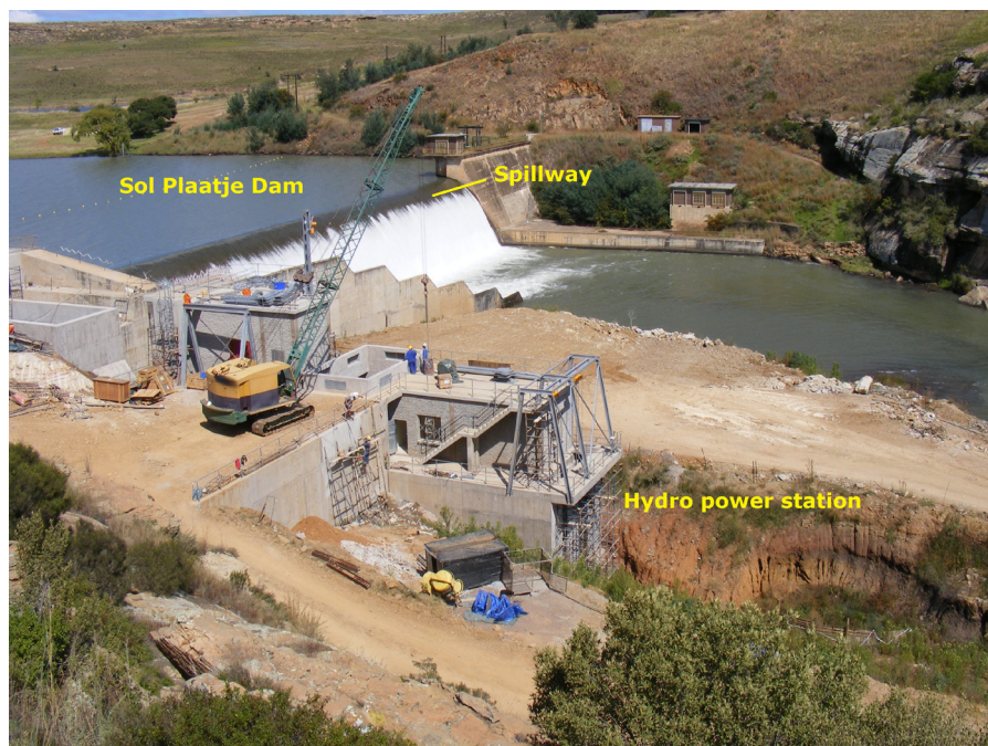
Figure 4 View of the Sol Plaatje Hydropower Project during construction
