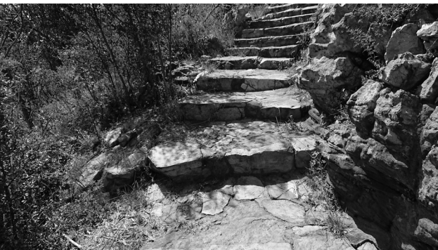
Fig.8.9 The Wilds Park: the use of natural stone, found on site, to construct dry-stacked retaining walls to articulate a pathway
