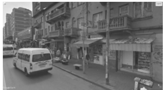
Fig.1.4 Dilapidated apartments and a degraded streetscape in Twist Street, Hillbrow (2018)
