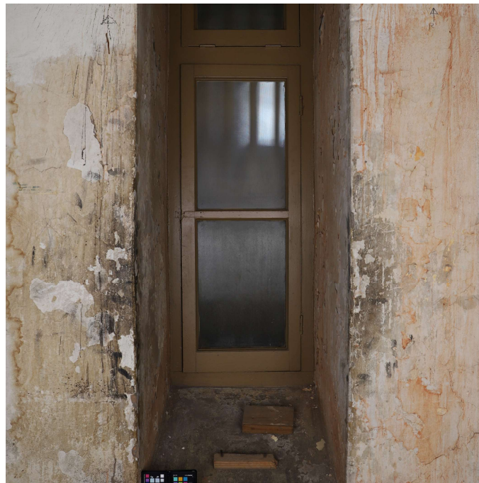
Figure 31: Fixtures on the North wall deep-seated window wall with iron nails. Photograph by author.
