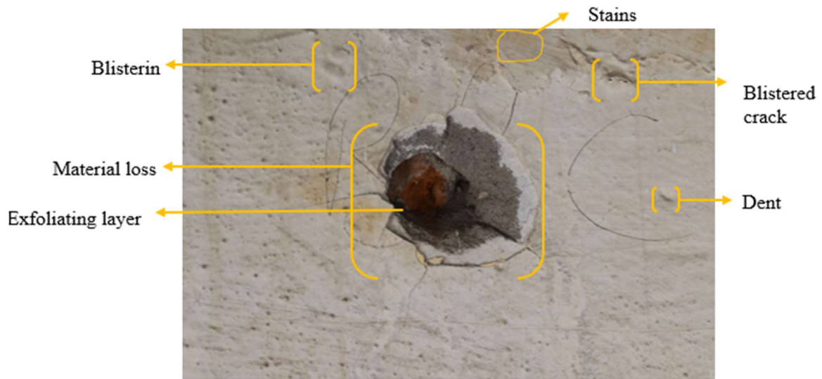
Figure 30: Wall strata on South wall lacuna. Photograph by author.
