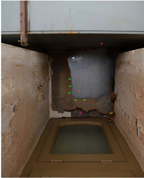
Figure 20: Ceiling material on North wall, above window. Photograph by author.
