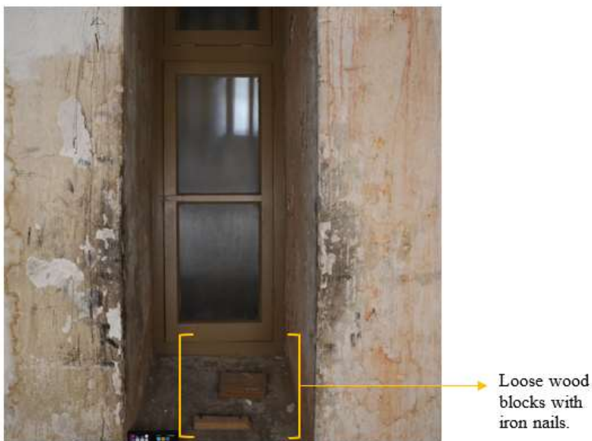
Figure 34: Fixtures on the North wall deep-seated window wall with iron nails. Photograph by author.
