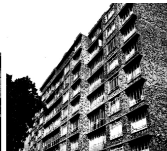
Fig.21 View of flat module in Erica Street [Author 2006]
