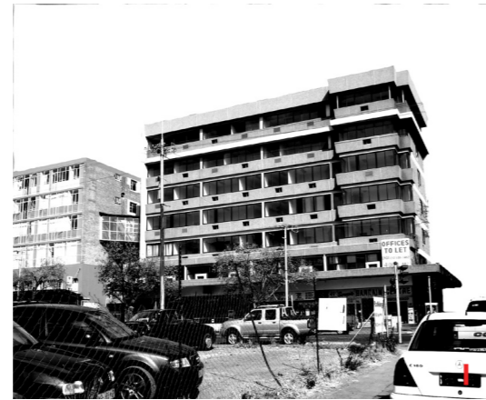
Fig.81 View of site from Mientjies Street [Author 2006]
