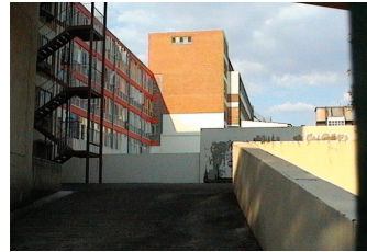
Fig.91 View towards Old police building parking bays [Author 2006]
