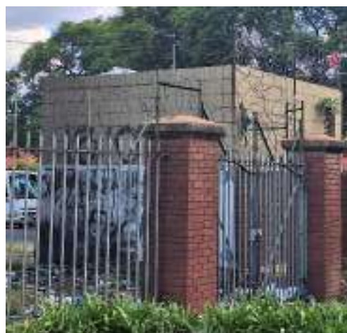
Figure 4: Fear-led design interventions - multi-fencing in Pretoria CBD
