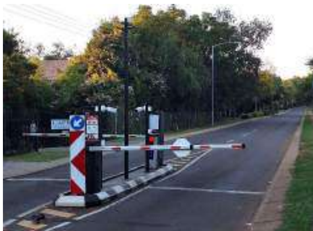
Figure 3: Access-controlled gated community in Lynnwood, City of Tshwane
