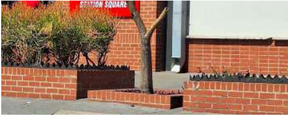
Figure 29: Anti-sitting spikes at the Station Square Mall
