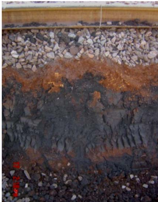
Figure 3-3: Overview of existing layerworks at the Amandelbult test section
