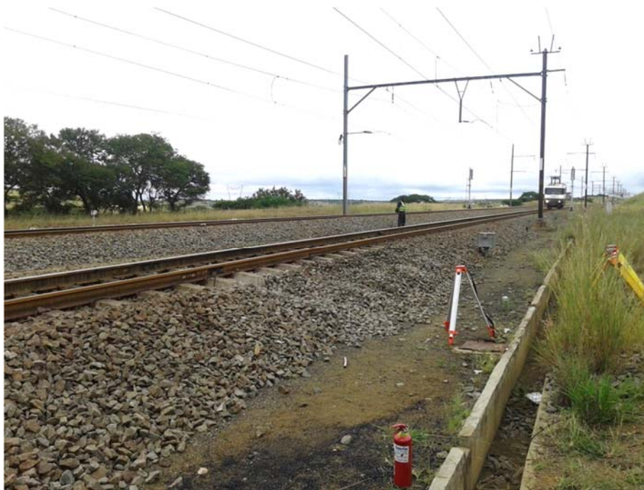
Figure 3-7: Overview of testing section at Bloubank
