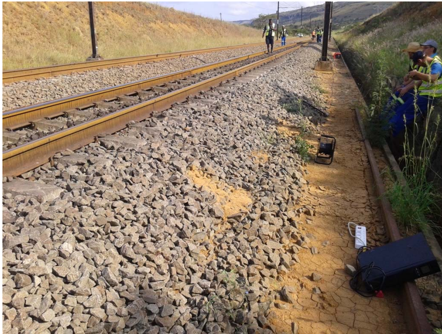
Figure 3-8: Izolof site at the start of testing (March 2015)
