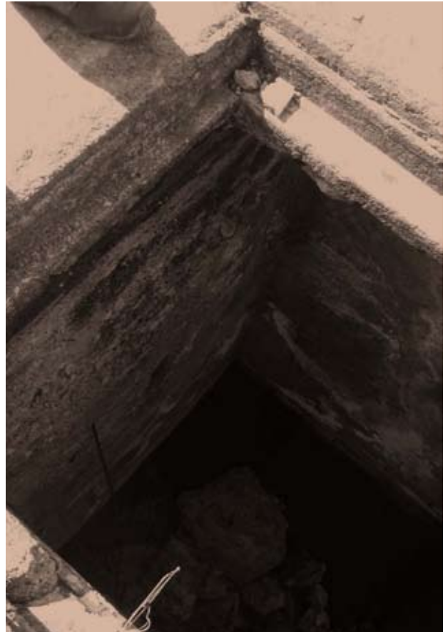
Figure 6.23 Existing storage tank with a depth of approximately 3m [August 2009]
