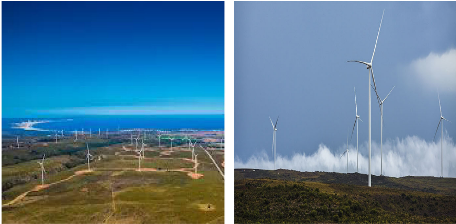
Fig. 1 Jeffreys Bay wind farm https://jeffreysbaywindfarm.co.za (left) and Noupoort wind farm https://noupoortwind.co.za (right)
