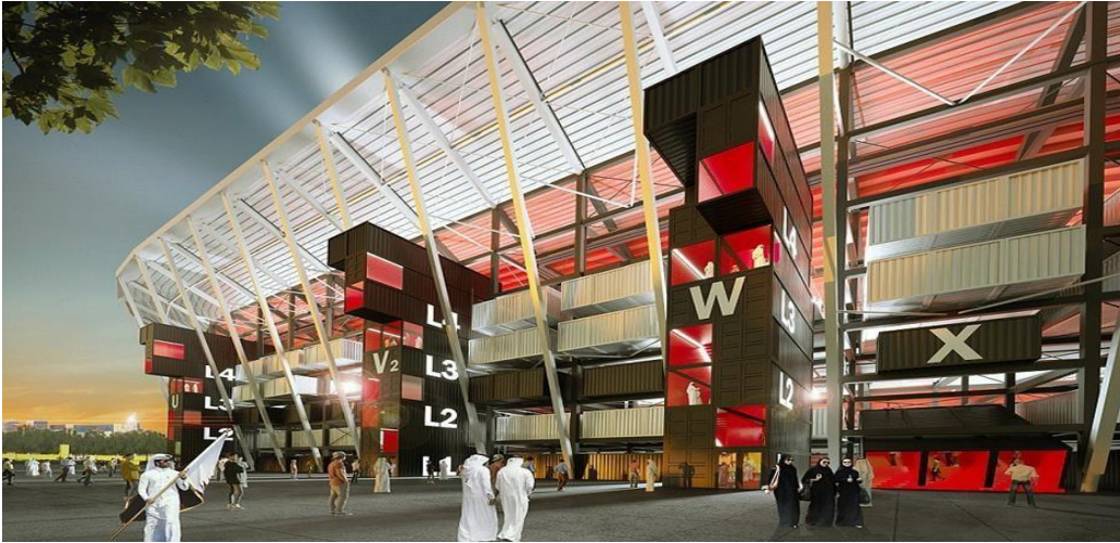
Figure 1: Digital illustration of the modified shipping containers and steel framework used to assemble the Ras Abu Aboud stadium
