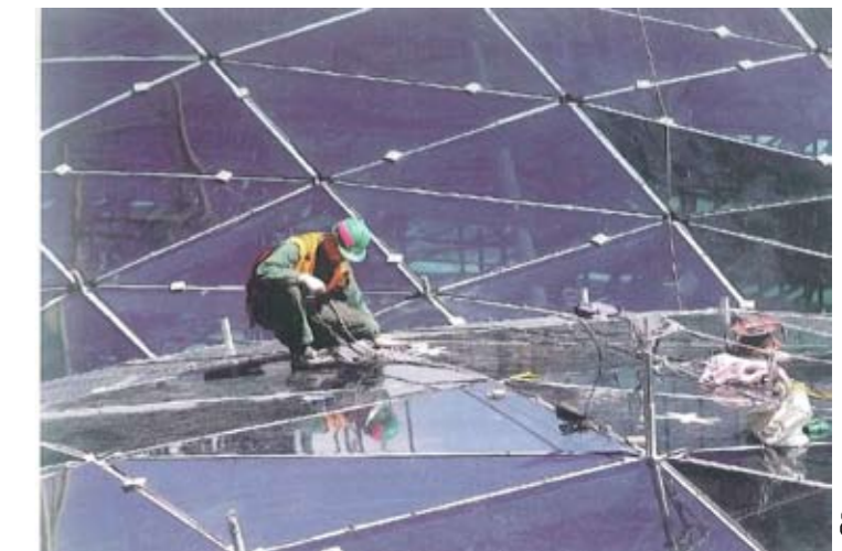
INSTALLATION OF GLAZING SEALANT
