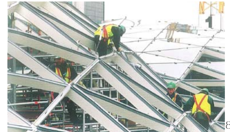
INSTALLATION OF GASKET SYSTEM
