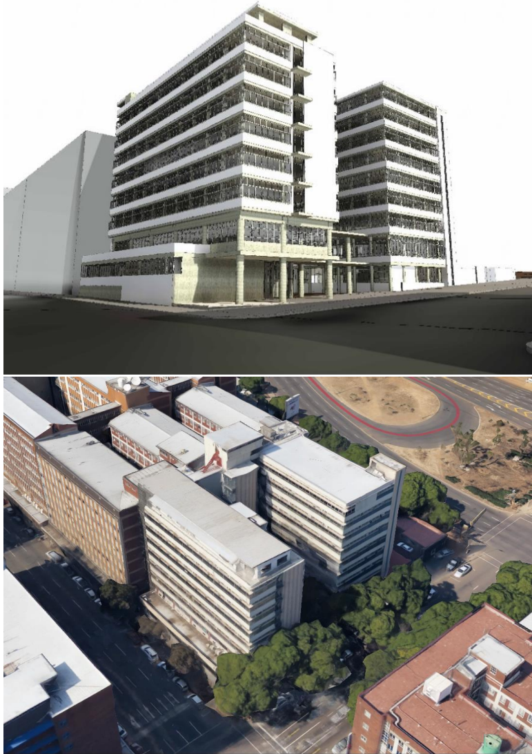
Figure 11: Revit Model Perspective of North and East Facade of the HB Philips Building (Top). Google Maps view of the North and East Facade of the HB Philips Building (Bottom)
