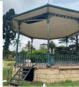
Figure 49: Current bandstand with Broken roof and balustrade, used for food donations.
