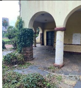
Figure 54: Current neglected and underutilised kiosk, where food was still sold after 2007.
