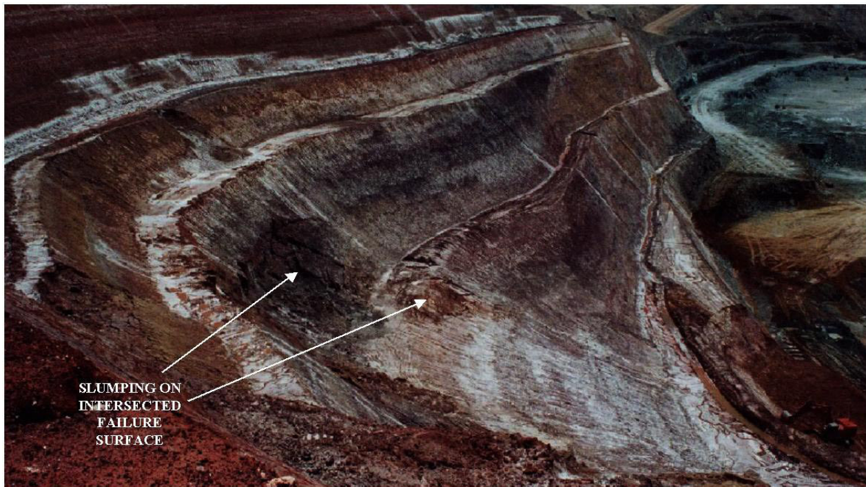
Figure 16: Remedial slope showing isolated slumping on old failure surface (Snowden, 2002)
