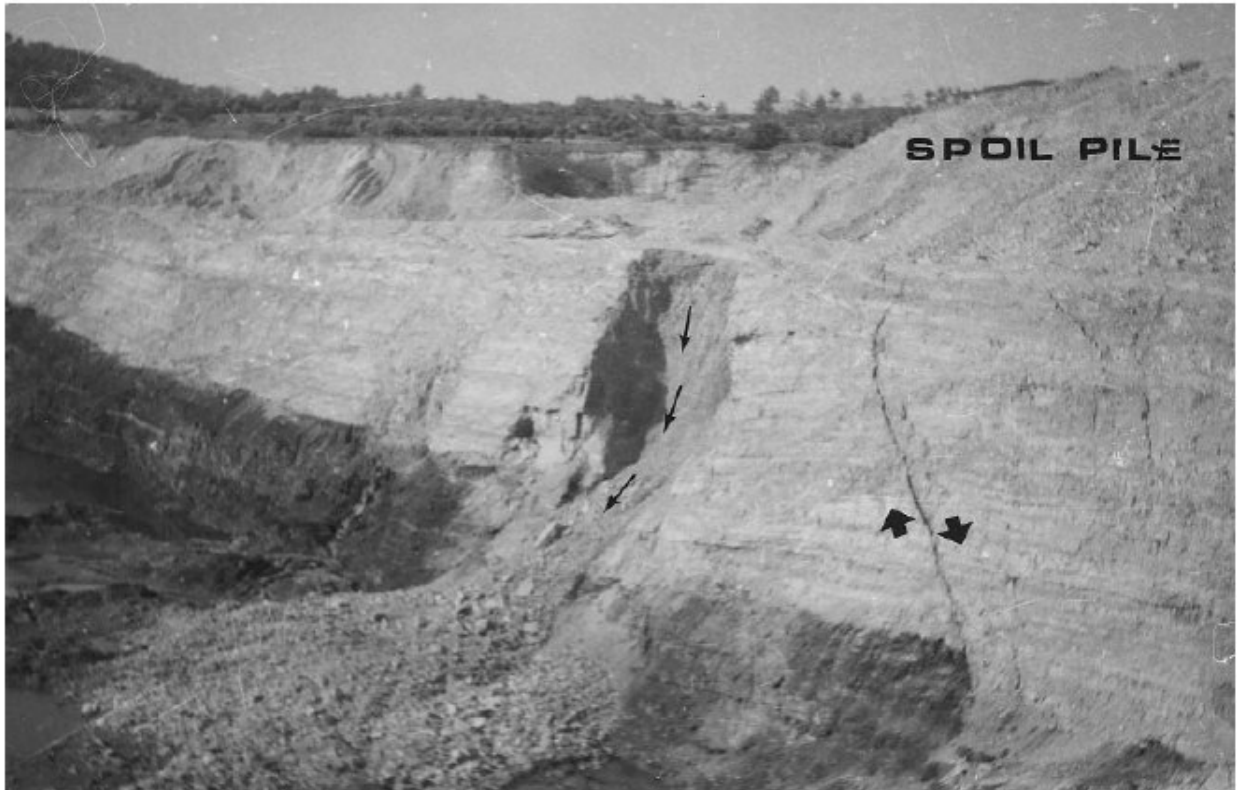
Figure 9: Initiation of the slide in the highwall externally loaded by a spoil (Sonmez et al., 1998)
