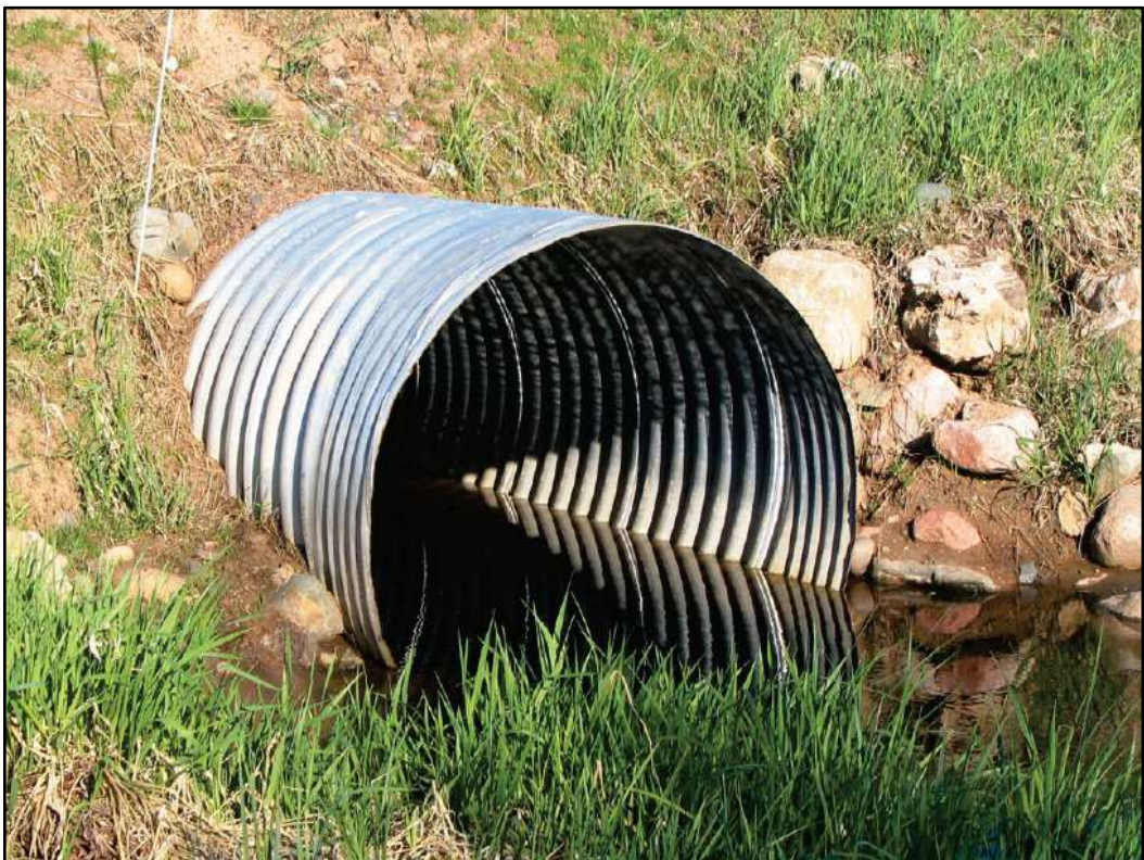
Figure 2-2: Corrugated metal pipe culvert (Schall et al. , 2012)
