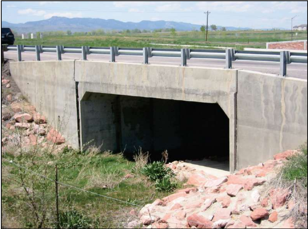
Figure 2-1: Concrete box culvert (Schall et al. , 2012)
