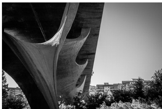
Figure 2: Basento river bridge (Luongo, 2016)
