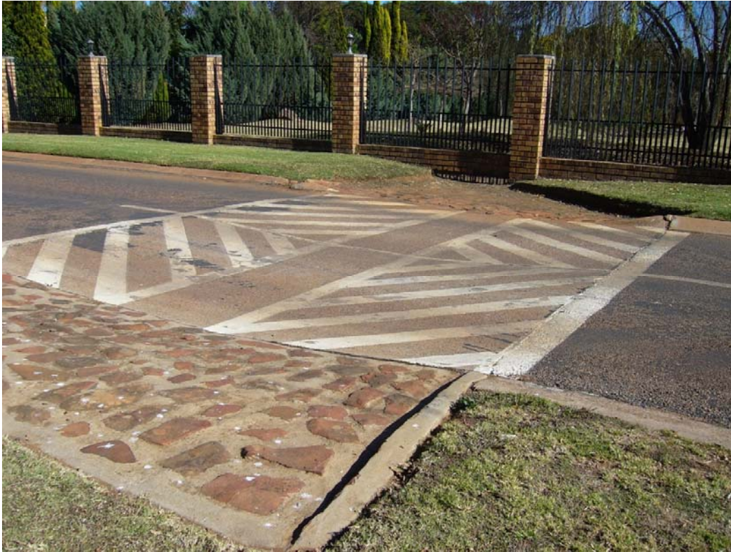
Figure 1. Example of a stormwater channel directing runoff from a street onto a residential property.
