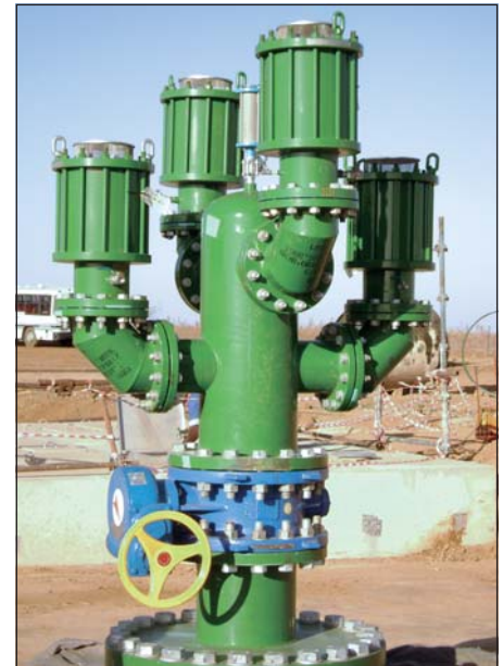
Figure 13 Air valve arrangement to ensure sequential closing and the provision of an air cushion
