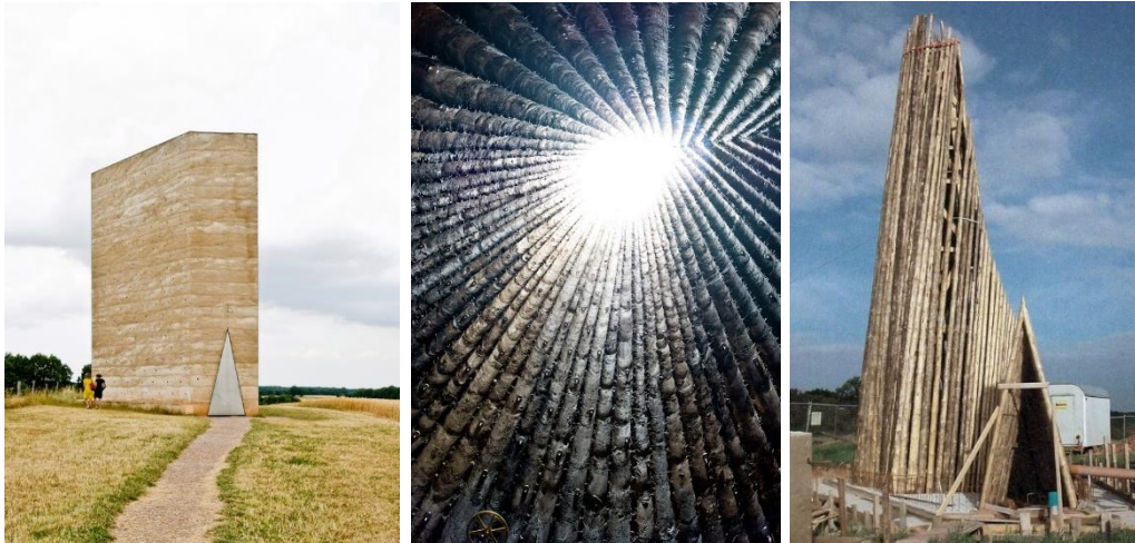
Figure 94. The exterior of the chapel is unassuming, yet the interior provides a different experience entirely. The 112 tree trunks were burnt after the concrete was cast (left) (archdaily.com)
