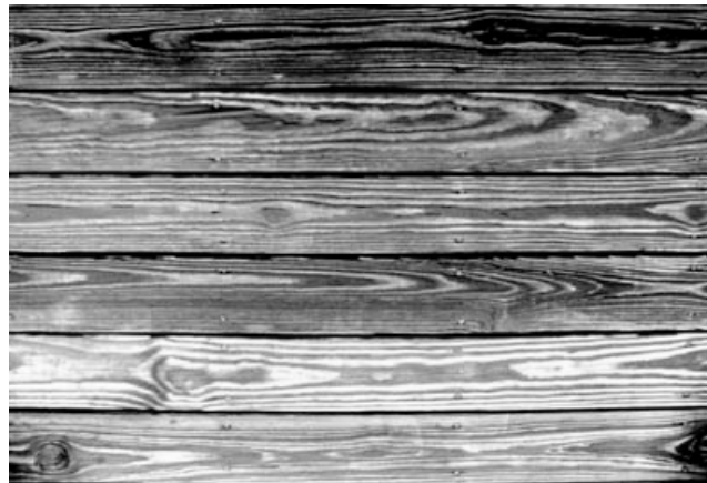
Fig 6.27 Timber is used for structure and cladding
