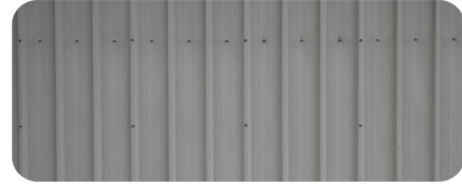
Concealed fix galvanised metal roof sheeting
