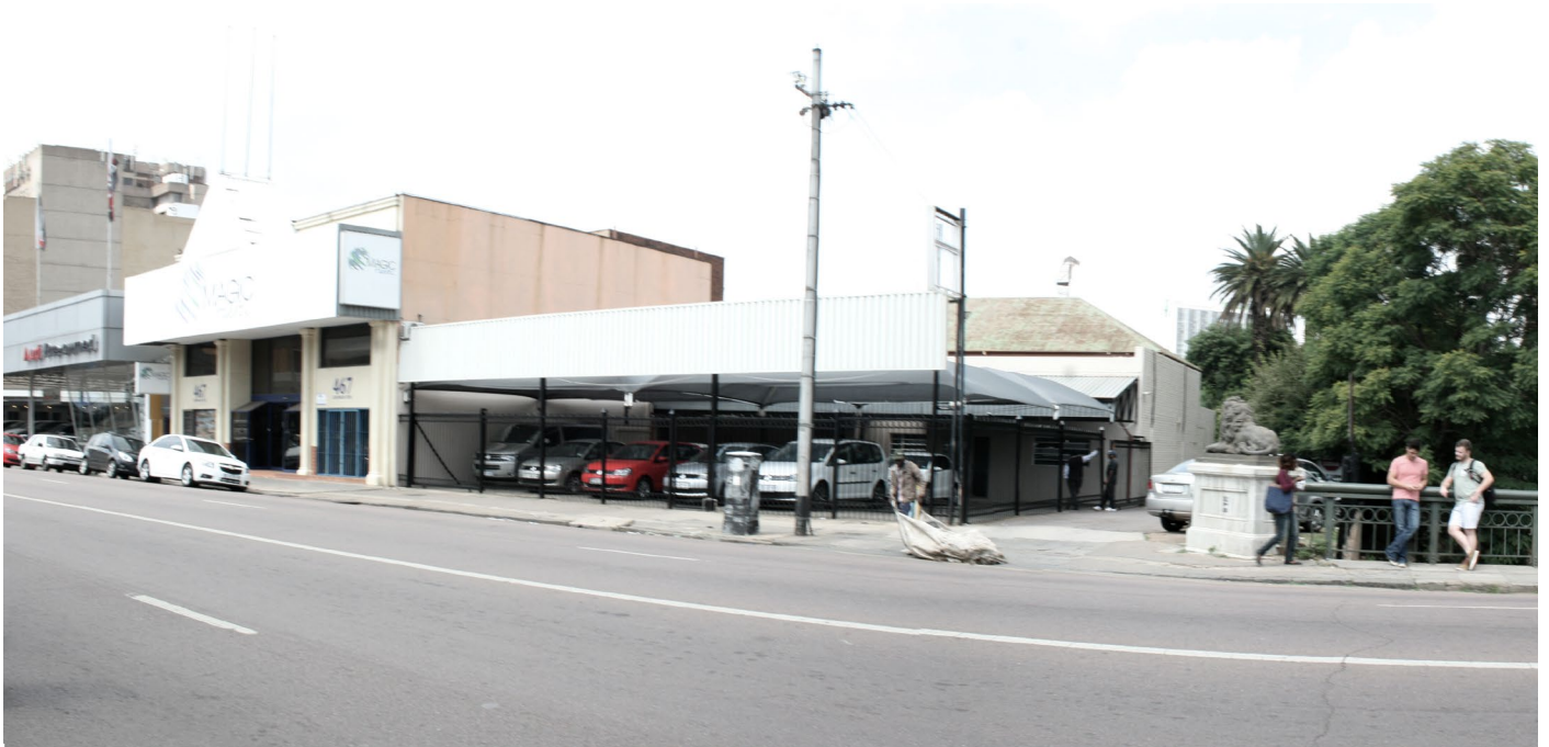
Figure 5.2: Panoramic view from Stanza Bopape street towards the site, Lion Bridge and the confluence of the Apies River and Walker Spruit. (Photograph by Author 2015)
