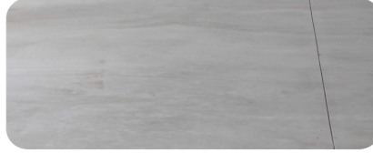
Steel trowelled finish to cast-in-situ reinforced concrete slabs
