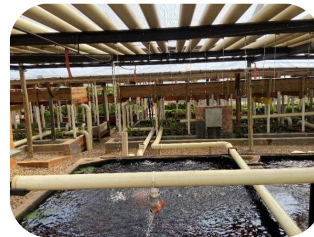
Figure 5.25-5.26: Illustrates the natural fall of pumped water breaking the surface of the water which is the only way oxygen is achieved in the fish tanks. Photo by Author 2021 (Author 2021).
