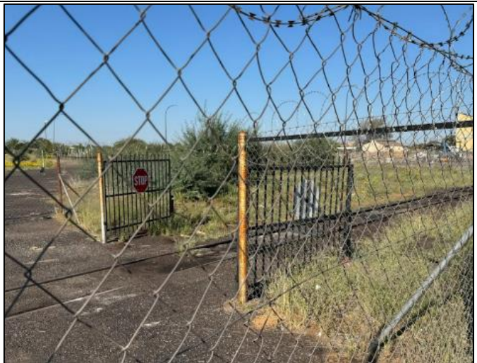
Figure 52 Railway infrastructure, (Source: Author,2024)
