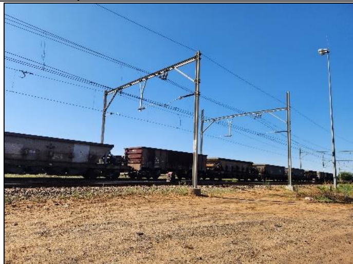
Figure 51 Railway infrastructure, (Source: Author,2024)
