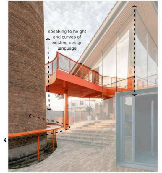
Contrast of materials and construction techniques that complement one another and showcase new vs old. New touches the old very lightly at specific connection points. New 'floats' around old or rests gently on it.
