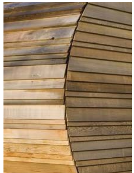
123. Sheep Stable - External Cladding Detail
