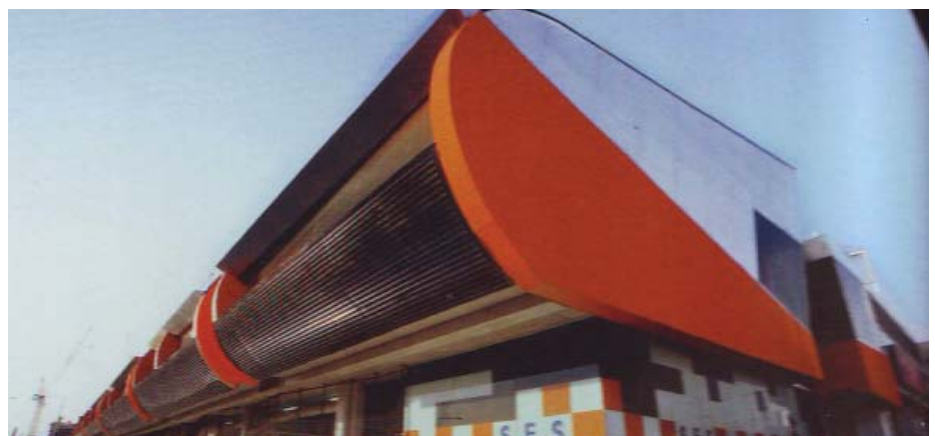
118. Emergency Services Headquarters - Fracturing and Colour Use
