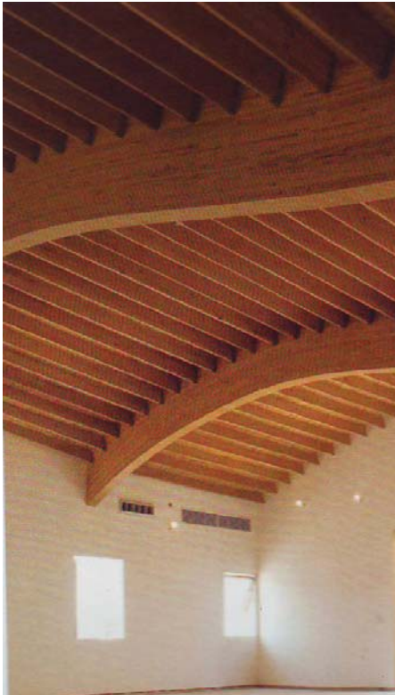
114. Commercial Building 3555 - Interior Ceiling
