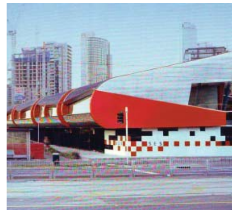
117. State Emergency Services Headquarters - View from Street
