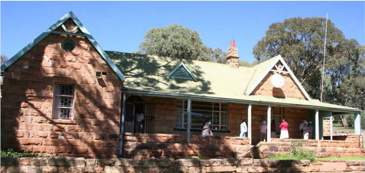
The Residency at Upper Moyeni where Masitise painted for How. The paintings are on the sandstone walls of the building, on the right hand side, under the verandah.
