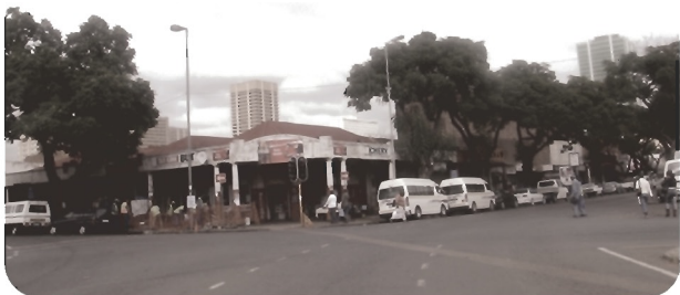
commercial building on the corner of bloed and prinsloo street
