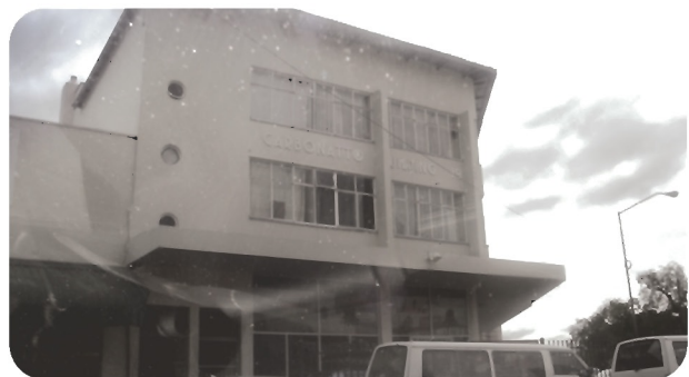
carbonatto building at dr. savage and boom street intersection
