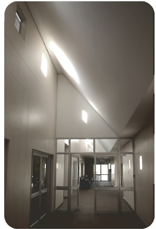
illus. 4.22 Clerestory windows with louvres in passage of the administration zone
