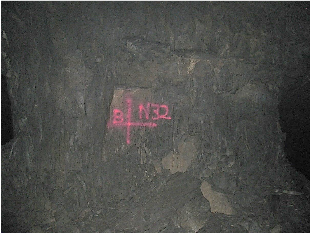
Figure 12-15. Side B of pillar N3_2 at Nchwaning III shaft as observed on the 18th of August 2021.
