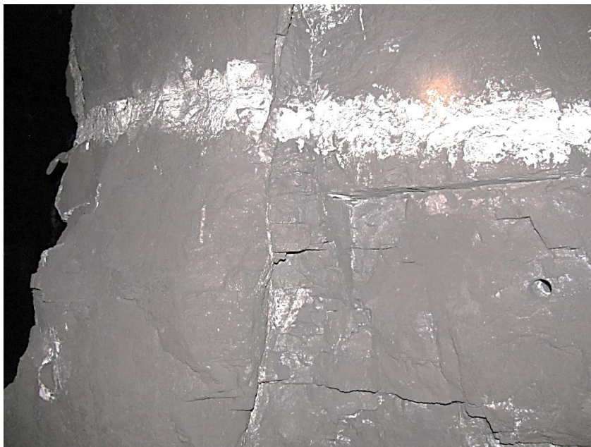
Figure 12-74. Side C of pillar N3_28 at Nchwane III shaft, illustrating the vertical and horizontal joint sets.
