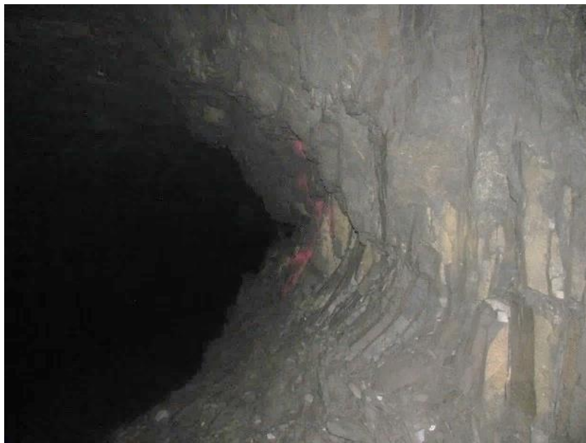
Figure 11-2. Depth of pillar scaling for pillar N3_1. Note the hourglass shape of the pillar.
