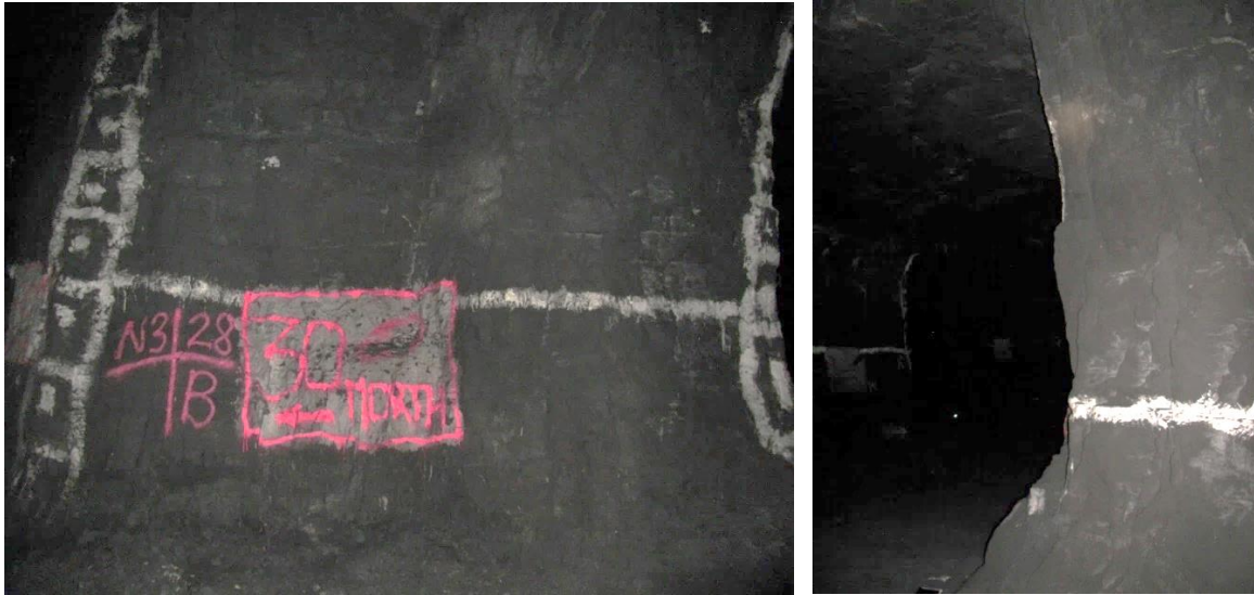
Figure 5-12. Typical condition of the pillars in Area 4. No scaling was observed.
