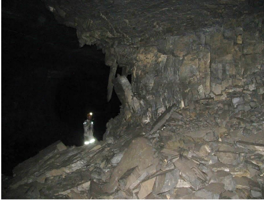
Figure 3-10. Extensive scaling of pillar N3_9.
