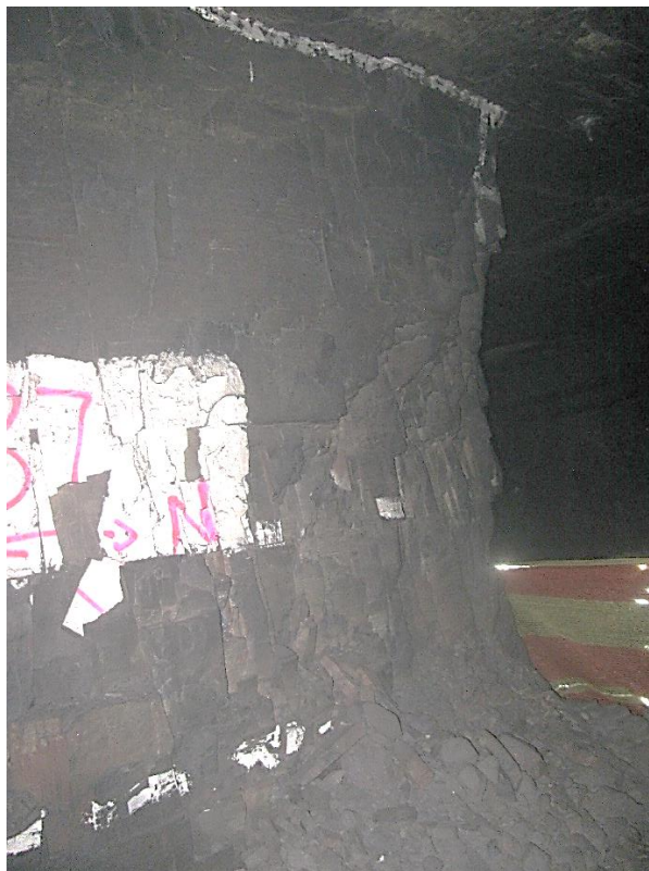
Figure 12-66. Side D of pillar N3_25 at Nchwaning III shaft, illustrating the right-hand corner of the pillar and no additional scaling of the corners was observed on the 18 th of August 2021.
