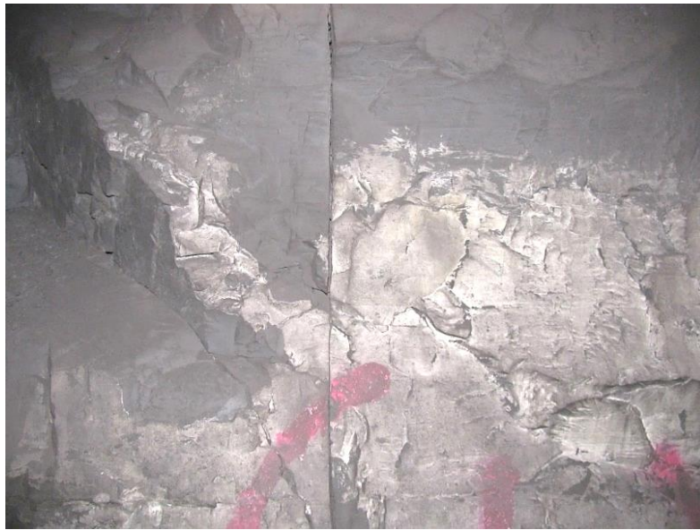
Figure 3-30. An illustration of the prominent vertical joint on sides A.
