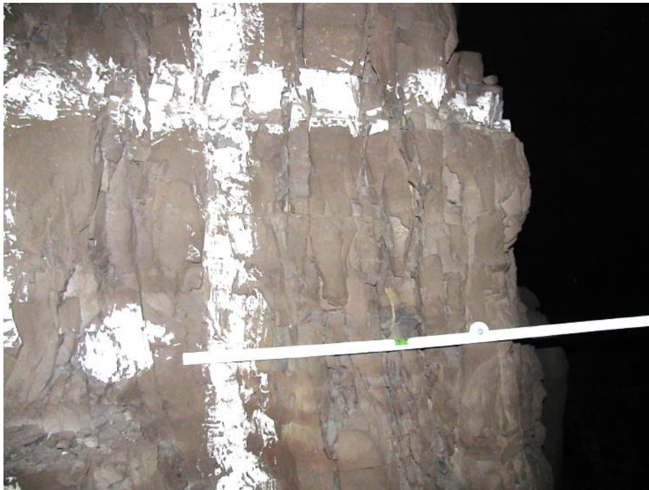
Figure 11-8. Side C illustrates the joint spacing, ranging from 5 cm to 20 cm.
