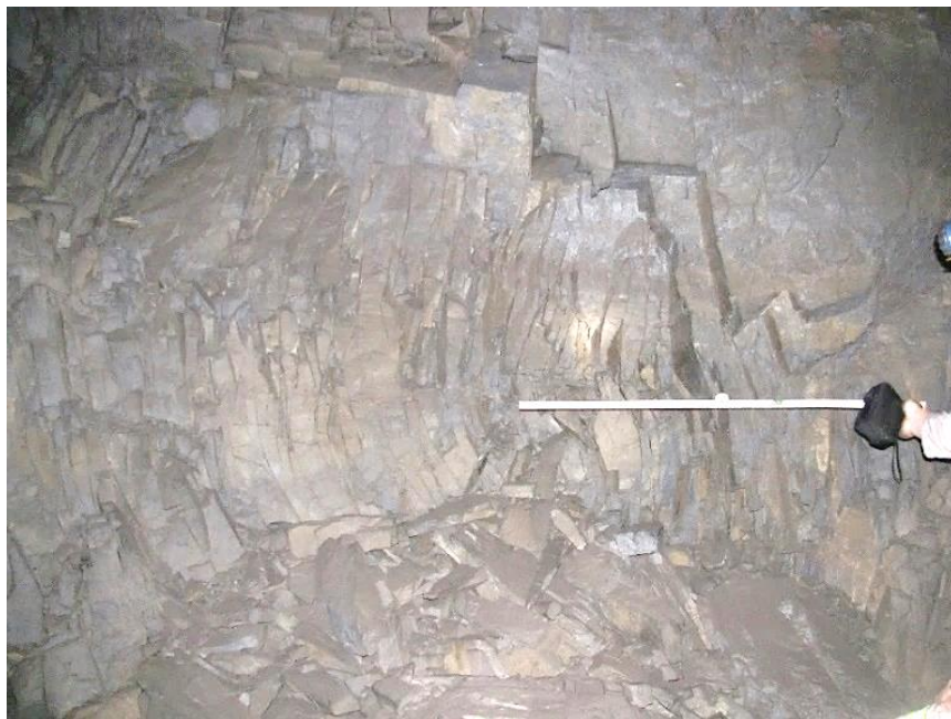
Figure 3-13. Spacing of the joints in pillar N3_9.
