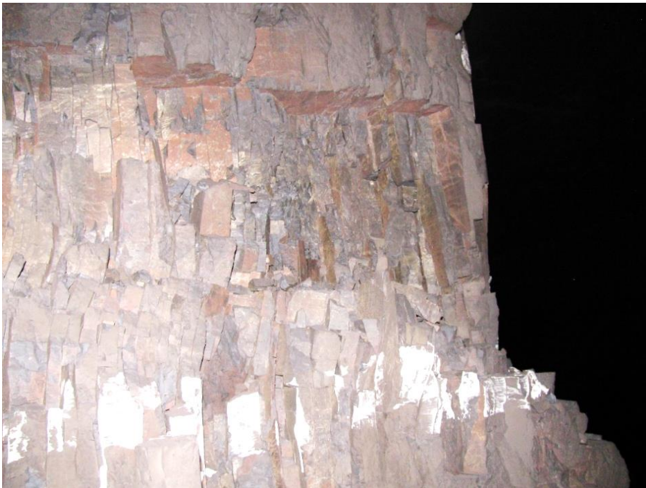
Figure 3-21. The vertical and horizontal joint spacing observed on side C of pillar N3_25. Note the varying joint spacing.
