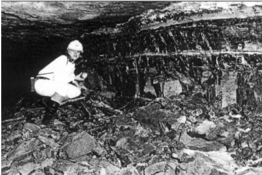
Figure 2-15. Ermelo B seam illustrating pillar scaling in a 90-year-old mining area (after Van der Merwe, 2003).
