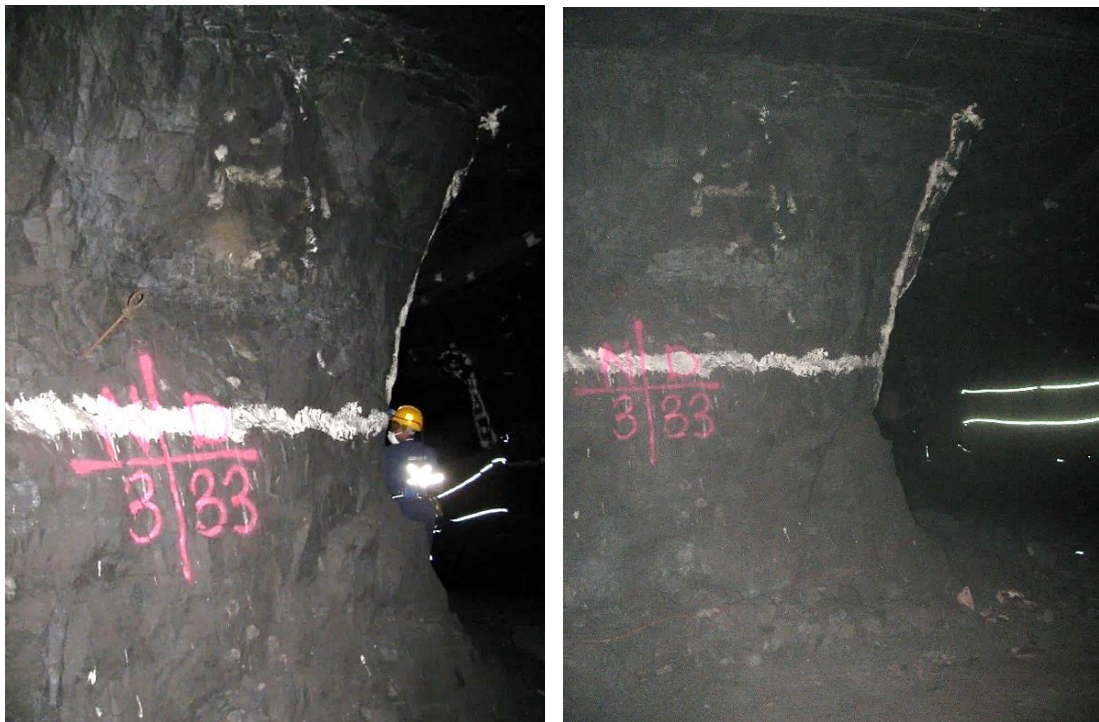
Figure 11-12. Side D of pillar N3_33 at Nchwane III shaft, illustrating the right-hand corner of the pillar observed on the 17 th of May and on the 18 th of August 2021.
