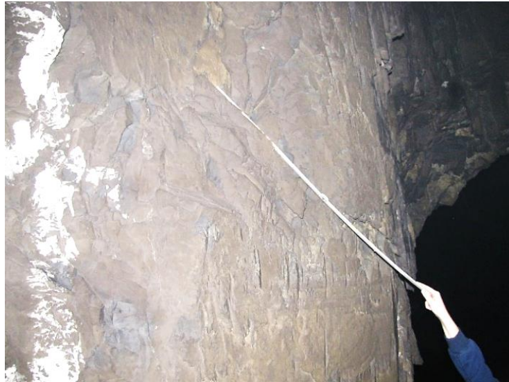
Figure 11-9. Random joint striking in the direction of Sides B and D. Angle of random joint, 45°.
