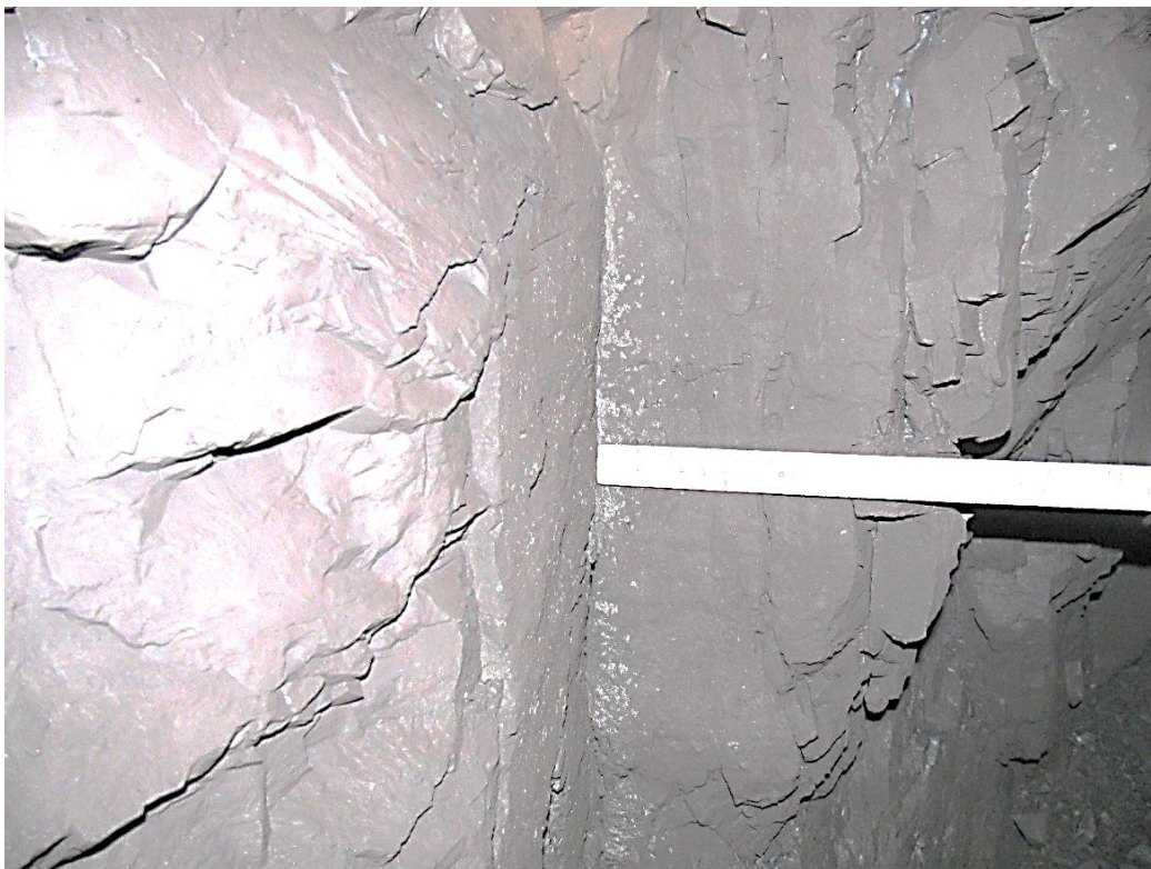
Figure 12-90. Side C of pillar N3_38 at Nchwaning III shaft, illustrating the vertical joint spacing on the edge of the pillar.
