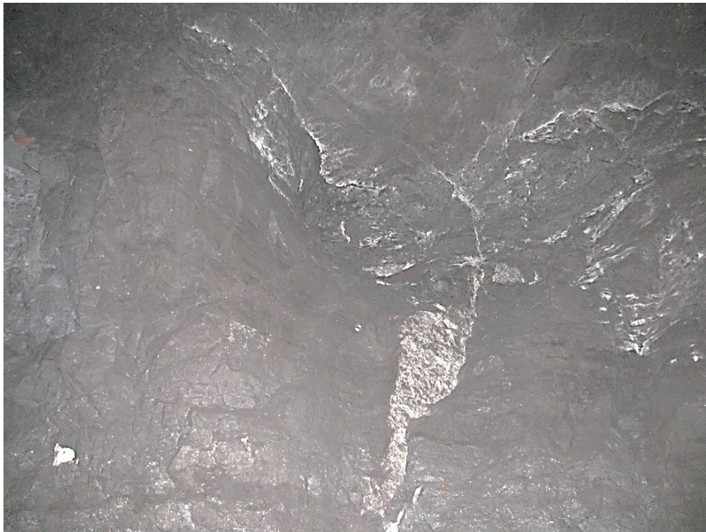
Figure 12-68. Side A of pillar N3_28 at Nchwane III shaft, illustrating the contact between the sidewall and the hanging wall.
