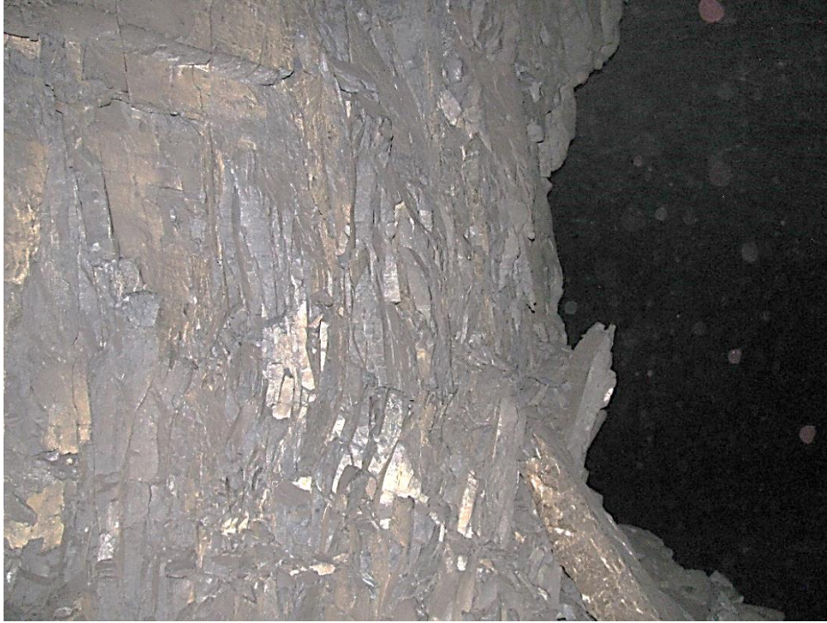
Figure 12-23. Side D of pillar N3_2 at Nchwane III shaft, illustrating the vertical joint sets on the right-hand corner of the pillar as observed on the 4 th of May 2021.
