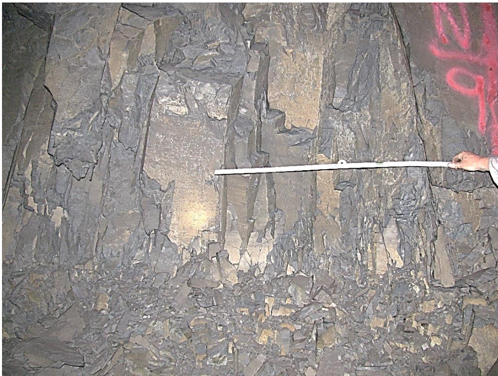
Figure 12-34. Side C of pillar N3_9 at Nchwaning III shaft, illustrating the vertical joint spacing on the left-hand side.
