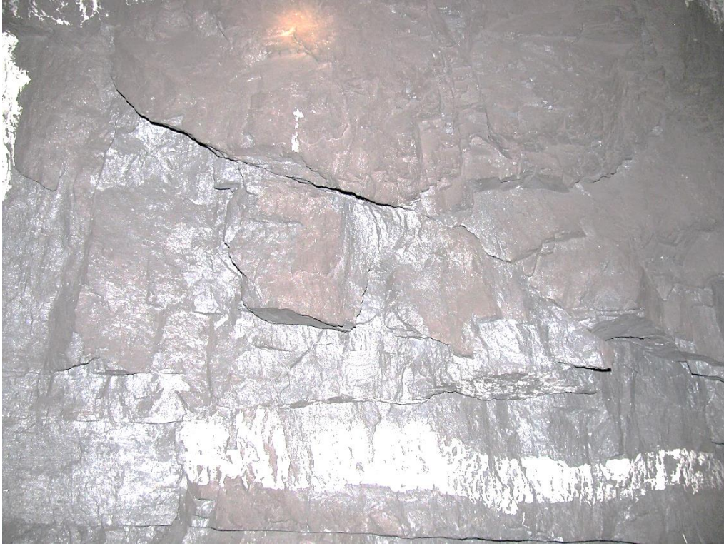
Figure 12-79. Side B of pillar N3_33 at Nchwaning III shaft, illustrating the horizontal joint set.
