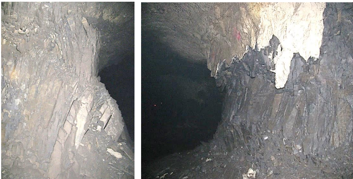
Figure 6-1. Example of pillar scaling at Nchwaning III shaft (left). This failure seems to occur in a time-dependent fashion. For the pillar on the right, a thin spray-on liner was applied to the pillar, but the scaling persisted and the liner failed.
