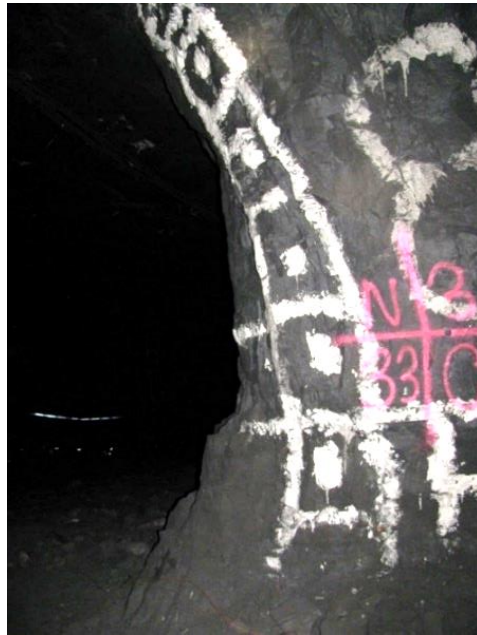
Figure 11-11. Side C illustrates an hourglass shape of the corners of the pillars. The pillar corners are still intact.
