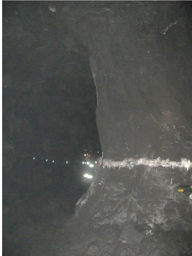
Figure 12-75. Side D of pillar N3_28 at Nchwaning III shaft, illustrating the left-hand corner of the pillar as observed on the 18th of August 2021.
