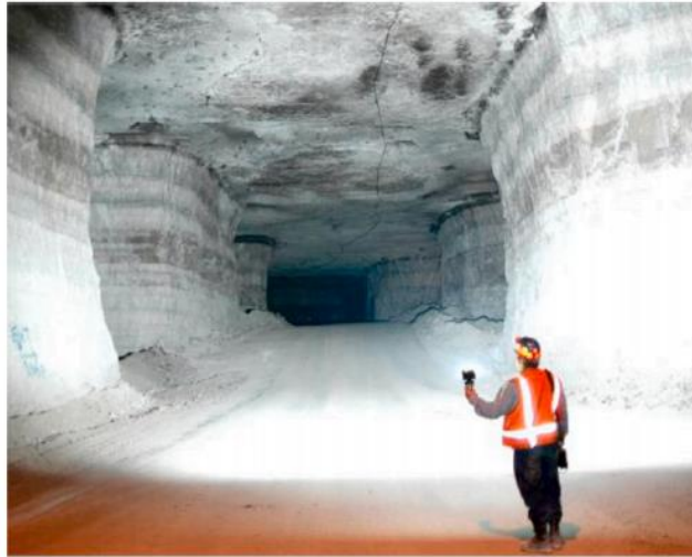
Figure 2-13. A stable limestone mine illustrating concave pillar geometry owing to time-dependent spalling damage (after Wang and Cai, 2021).
