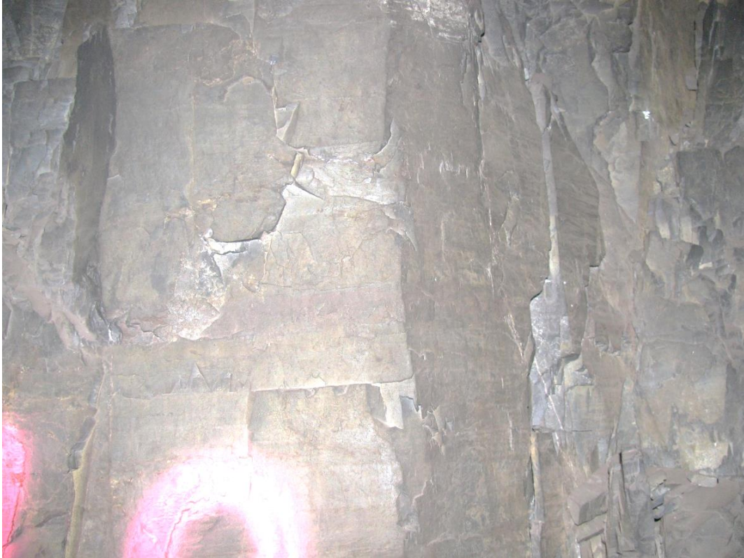
Figure 12-55. Side D of pillar N3_20 at Nchwane III shaft, illustrating the two joint sets.
