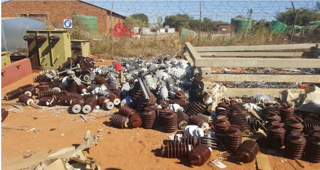
Figure 4.9: Insulators, scrap conductors & defective transformers placed on the ground, Kwaggafontein CNC – Emalahleni Zone
