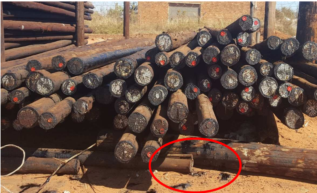
Figure 4.12: Wooden poles with creosote wearing off the poles, Kwaggafontein CNC – Emalahleni Zone (Source: Author's Own)
