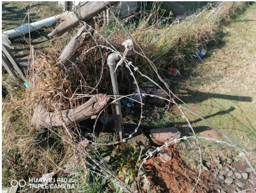
Photo P5(1): Environmental risk: Leaking water tap not being fixed
