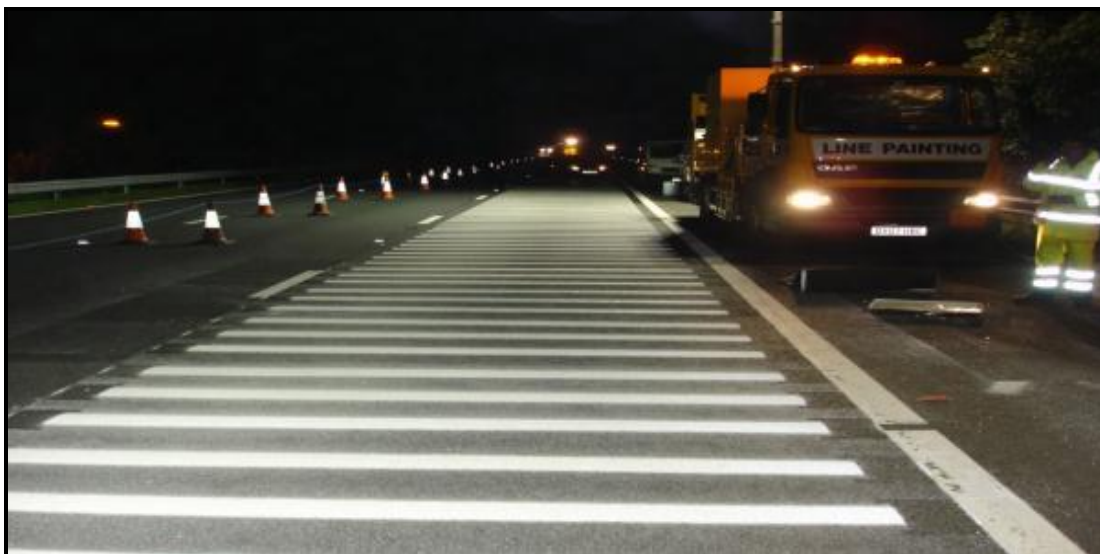
Figure 2.2: Road trial of road markings in the UK (Europe) (Owen, 2013).
