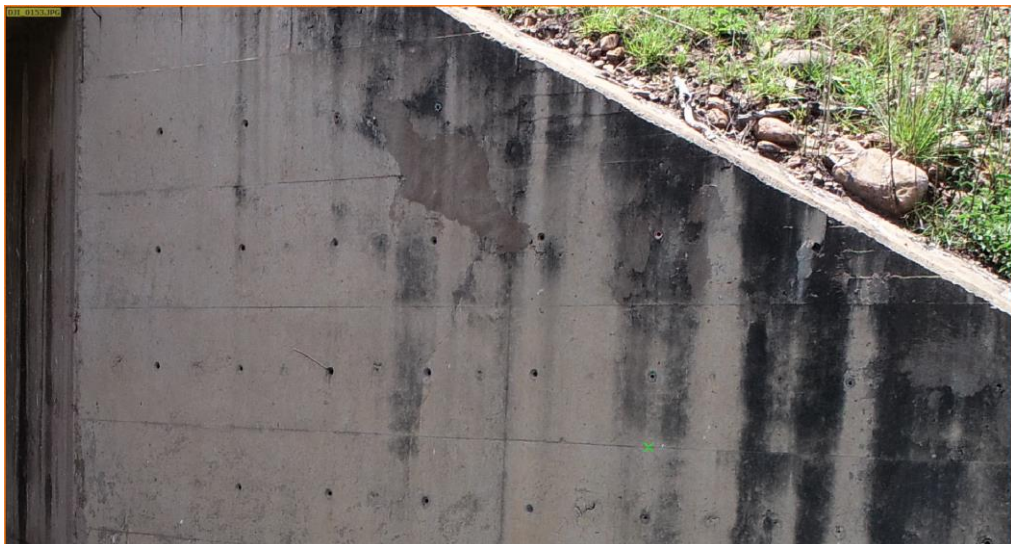
Figure 3-10: Enlarged image of the selected bridge element
