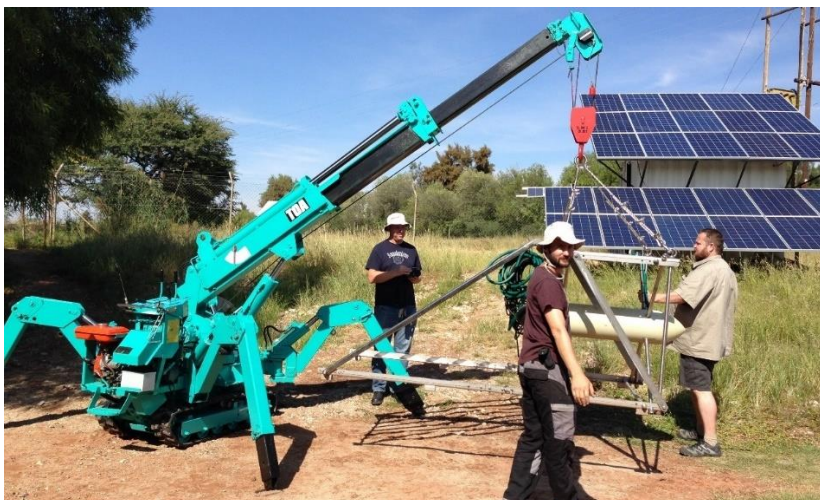
Figure A-7: TOA Crawler crane
