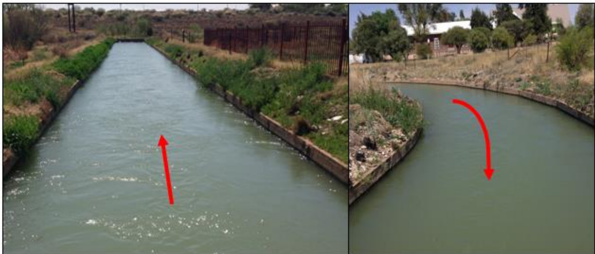
Figure 3-18: Canal system at the Groblershoop site
