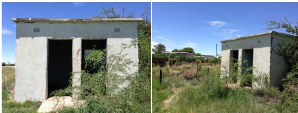
Figure 3-16: Existing pump station building
