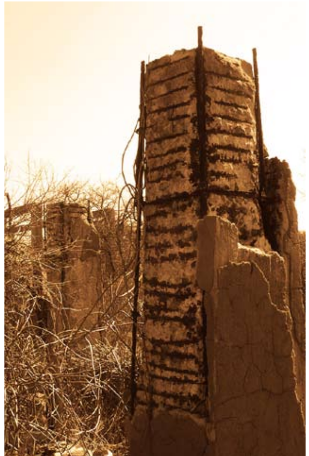
Figure 5.23 Reinforced concrete column structure [March 2009]
