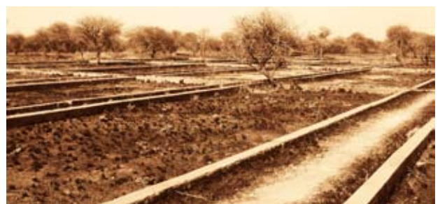
Figure 5.24 Foundations of historic warming ponds [August 2009]
