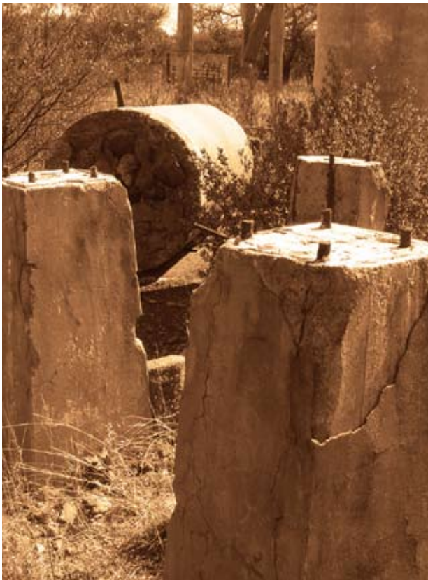
Figure 5.21 Reinforced concrete elements [March 2009]
