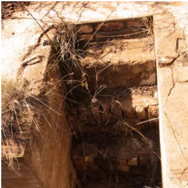
Figure 5.16 Small stairs leading into open storage tank [March 2009]
