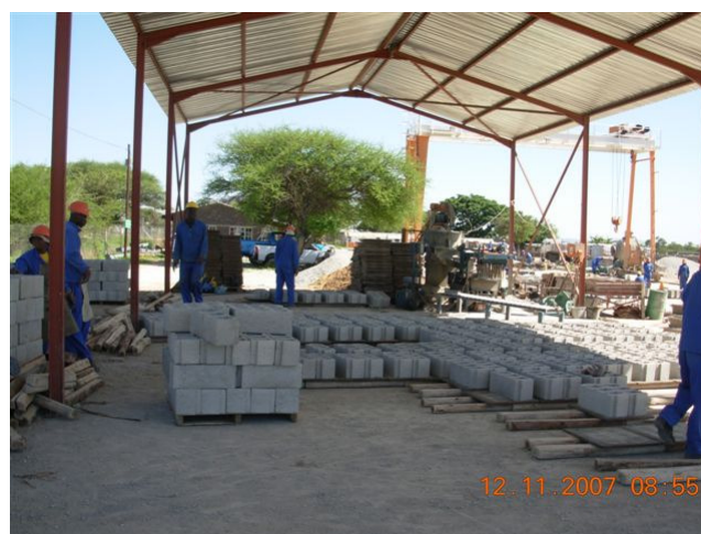
Figure 26 - Block Production Shed
