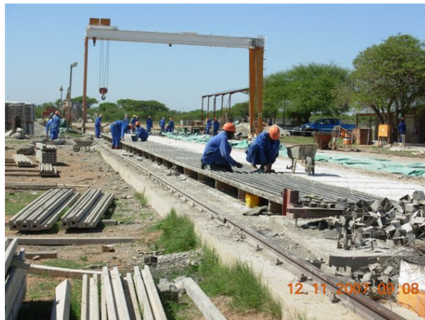
Figure 28 - Lintel Labourers Kneeling
