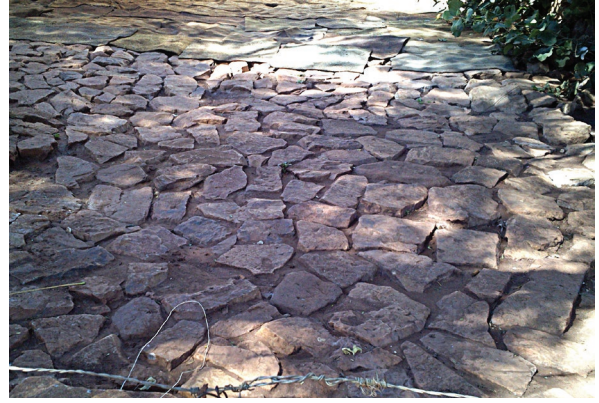
Figure 49 Existing stone surface skills in Alaska (Author 2015)
