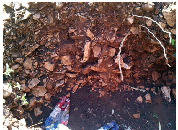
Figure 26 Abandoned hole dug in preparation for pit latrine exposes rocky nature of soil (Author 2015)
