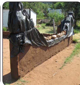
MUD PLASTERED ROCK WALL
