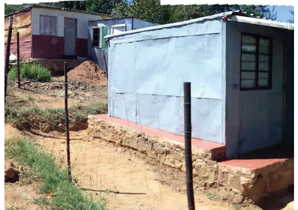
Figure 27 Houses on plinths built on cut & fill sections. Plinths double as seating (Author 2015)
