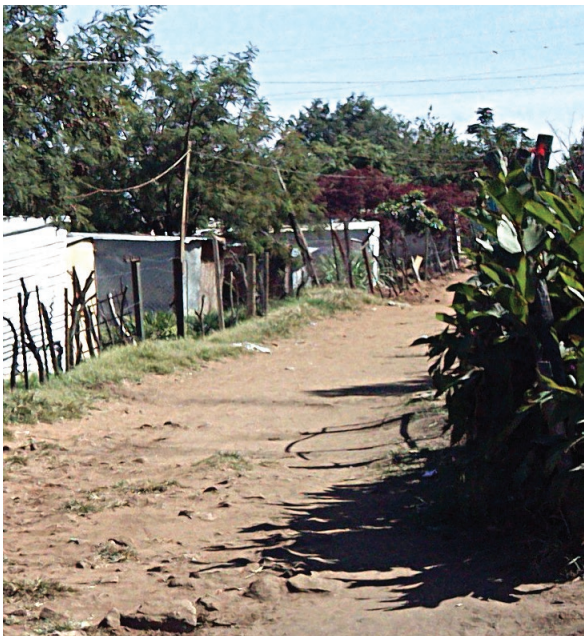
Figure 25 Much less erosion from roads running perpendicular to the mountain's slope (Author 2015)
