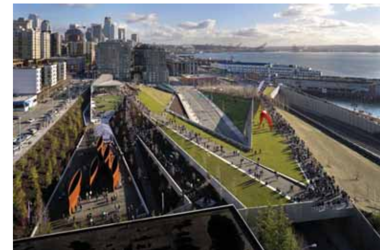
Figure 5.35. Pedestrians using the z-shaped path that traverses above vehicular traffic. (Detail, 2010)
