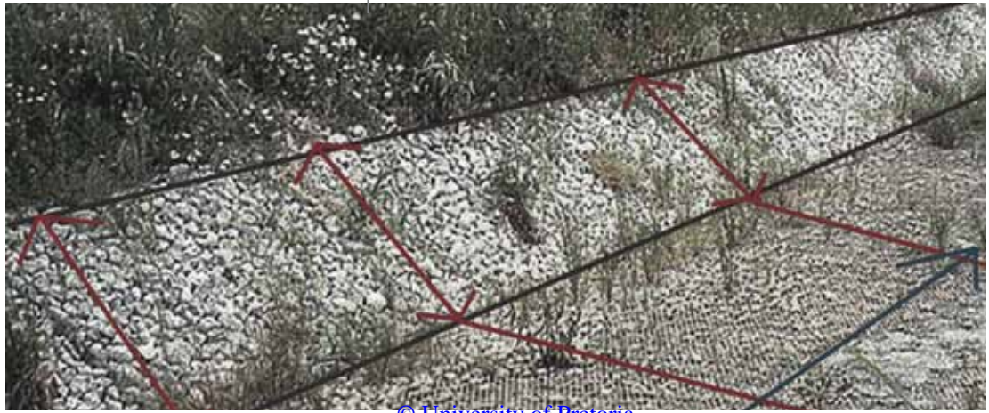
Figure 57: Reno Mattress Stream Rehabilitation Rock packed reno mattresses are used to line stormwater channels ( www.koboxvizpartvedelem.hu )
