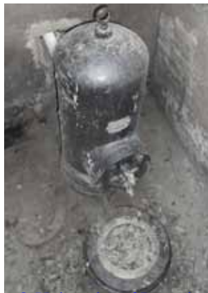
Figure 59: Hydraulic ram Functioning hydraulic ram on Schutte Farm (Author: 2012)
