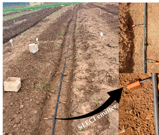
Figure 2. Subsurface Low-Energy Clay Irrigation line and installation of tubes.
