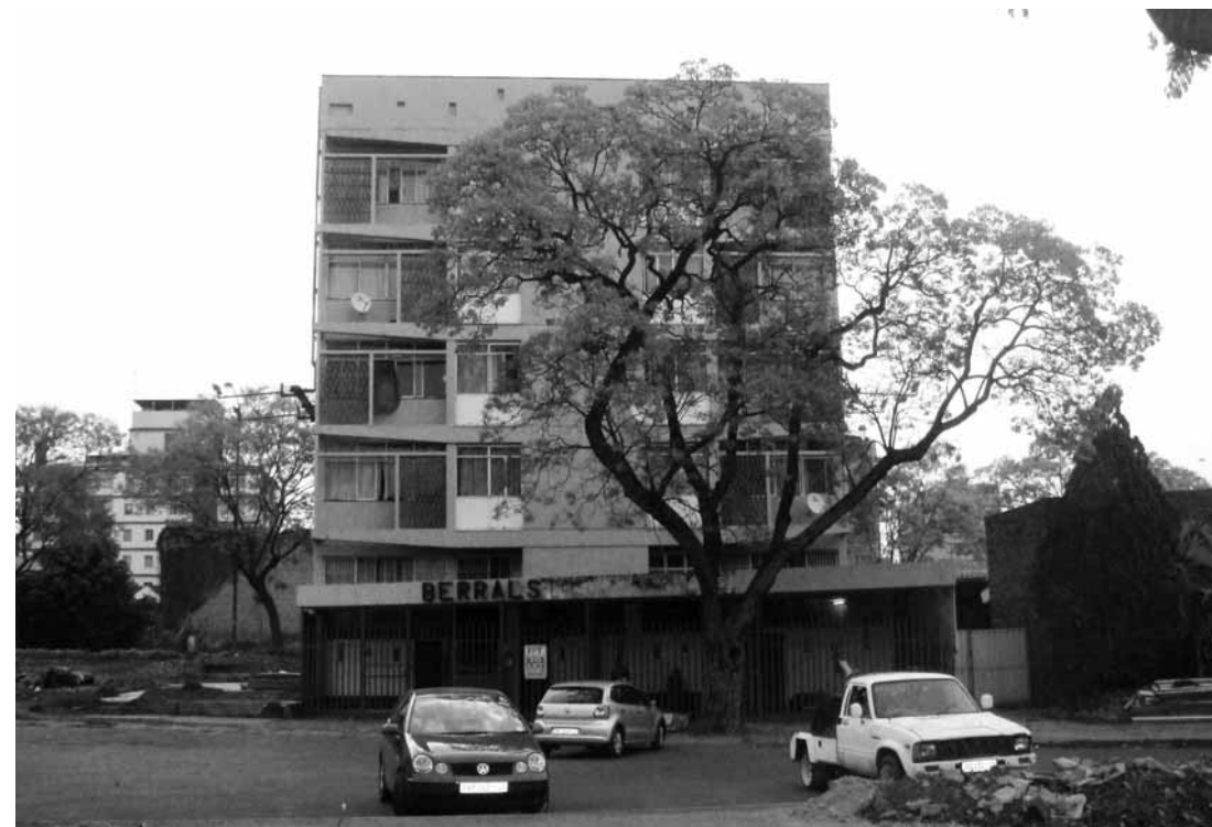
Figure 6.38. (below) The Berrals building - Eastern facade with the brise soleil screen (Author, 2010)
