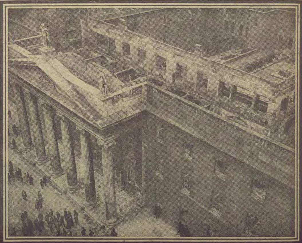
A view of the wrecked General Post Office. Only the portico and outer walls remain.
