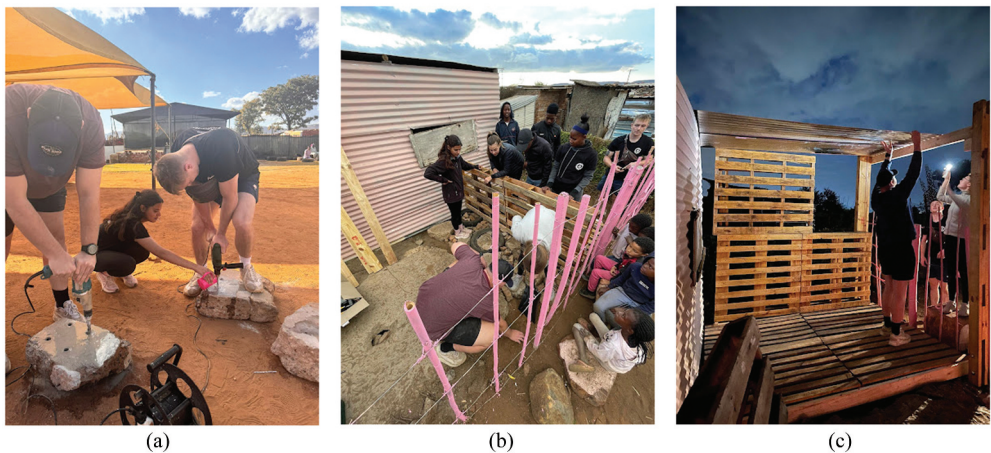
Figure 10. Hands-on workshops and live build in the informal settlement.
