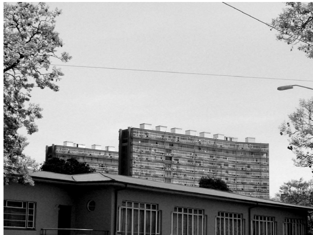
Figure 66 (top) View looking south- west towards site from the Pretoria Art Mu- seum. Author, 2006
