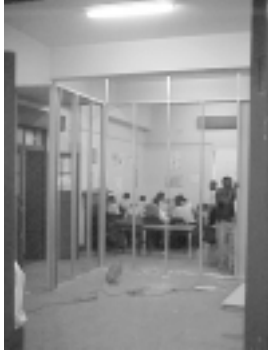
Figure 6.10: South Clubhouse, refurbishing of new classrooms
