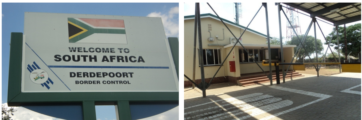
Figure 4 Derdepoort border post
