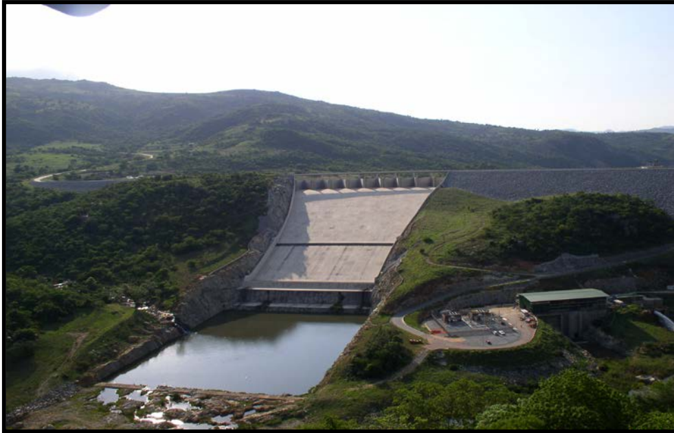
Figure 4.12: Maguga dam with hydropower plant on the right Source: ICMA (2010)
