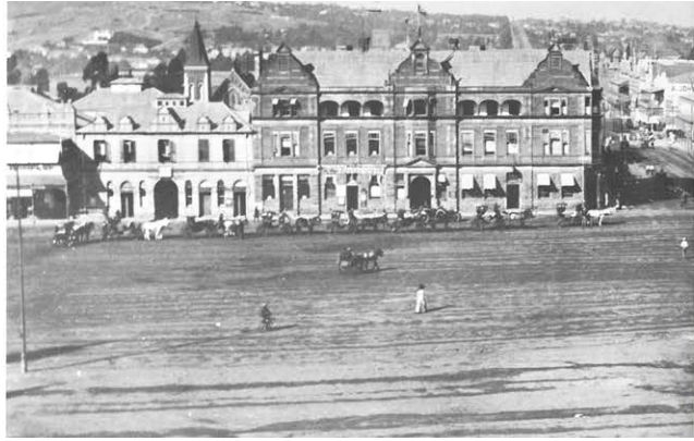
Figure 55: Church Square 1905, Slow place (Vivien Allen, 2018)
