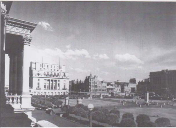
Figure 61: Church Square from Standard Bank building 1934 (Friedel Hansen, 2018)
