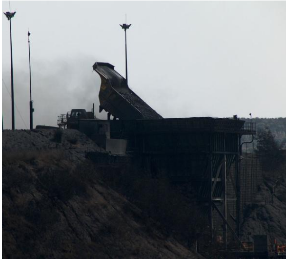
Figure 8: Truck Offloading at Tip Bin
