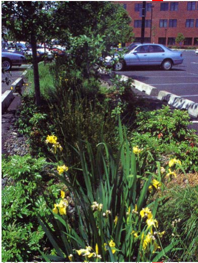
2.17. In Portland traditional sidewalk planting is being replaced by a series of interconnected swales which act as stormwater treatment cells which intercept and filter street runoff (Owens Viani 2005)
