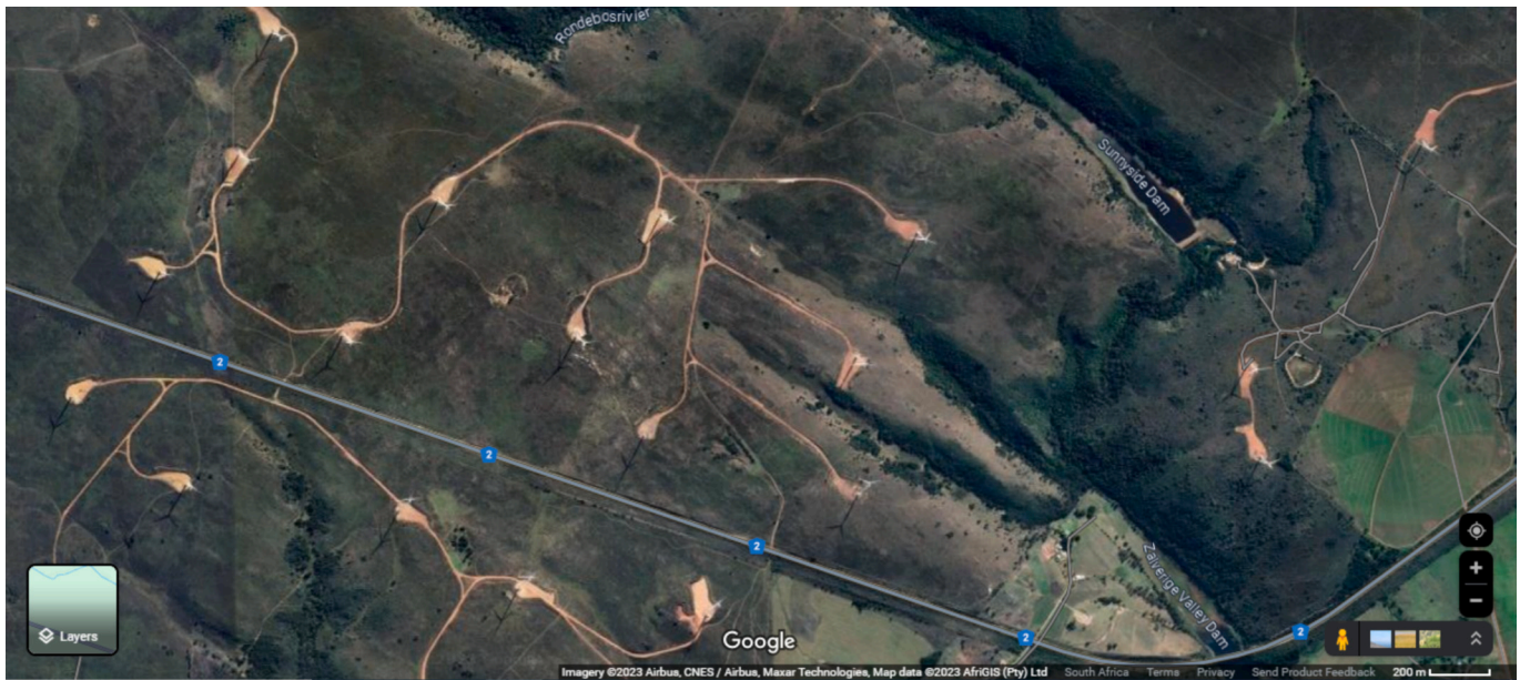
Fig. 1. Jeffreys bay wind farm location [80].
